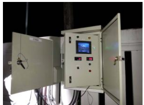
Fig. 1-2: Enclosure panel with the Expert Remote I/O module and Industry Expert Panel PC and Power Switch and UPS and Wire connection
