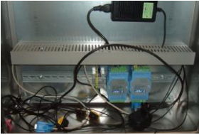
Fig. 2-3 : Wire connection for Expert Remote I/O module in Enclosure of Control Panel
