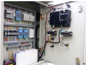
Fig. 1-1: Separated the Expert Remote I/O module and Industry Expert Panel PC
